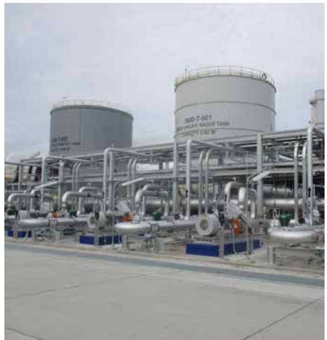
PTTLNG Cold Water Generation Plant (EPC)
