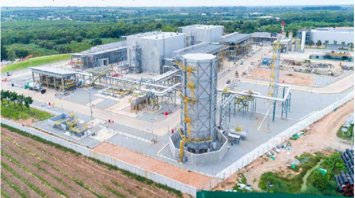
PTT Midline Compressor Station (SMP / E&I)
