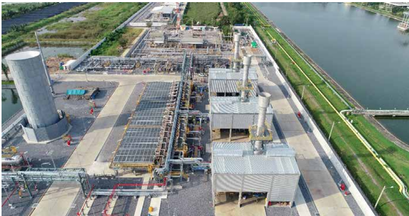
PTT Wangnoi Compressor Station (Civil & SMP)
